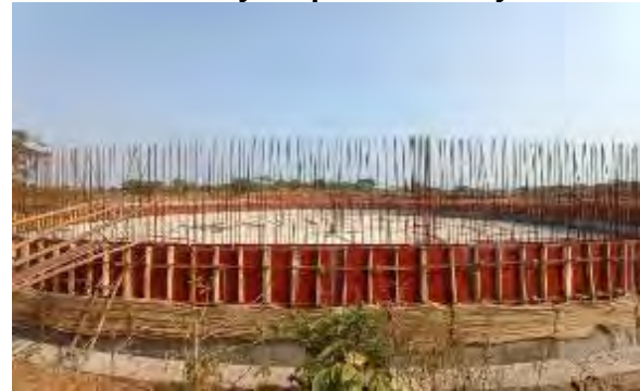
Clariflocculator 2 at WTP under construction
