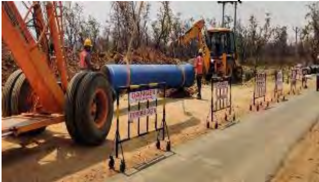
Pipe laying Activity at Supur More
