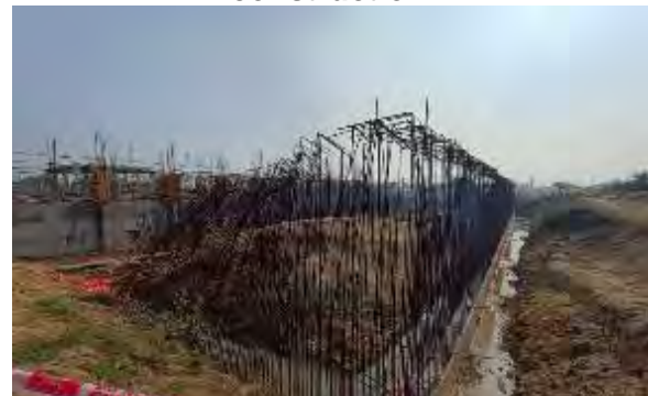
Gobindpur GLSR under construction
