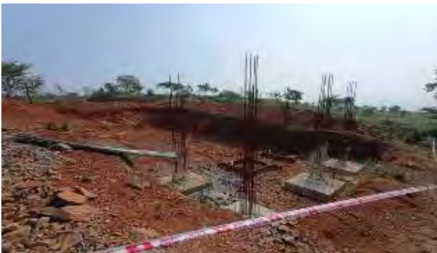
Staff Quarters under construction
