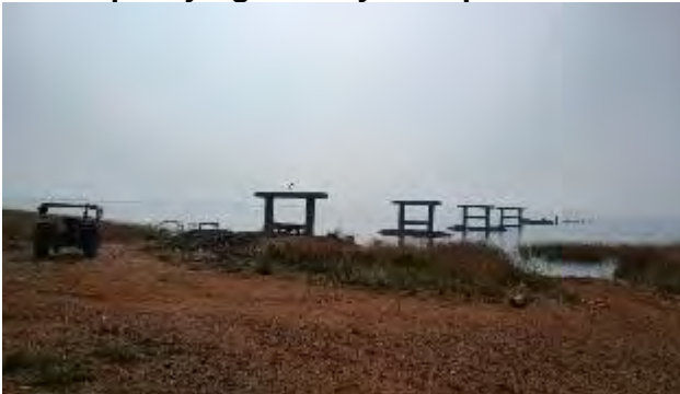
Intake approach bridge under construction
