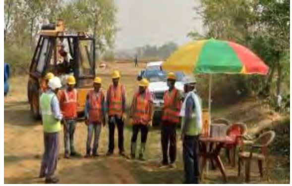
Tool box talk at pipe laying site
