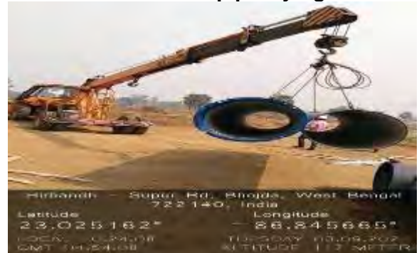
Third Party Inspection of Hydra
